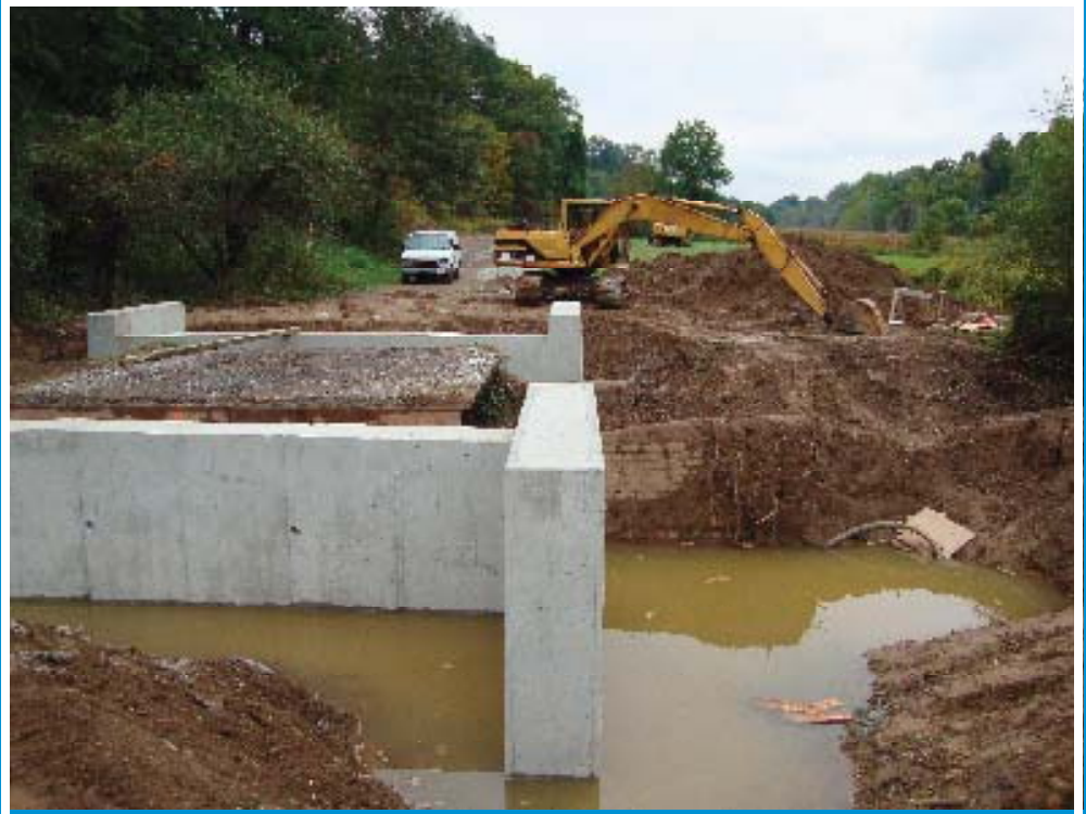
Picture above shows work being completed on Sugar Camp-Jackson Fork Road Bridge
