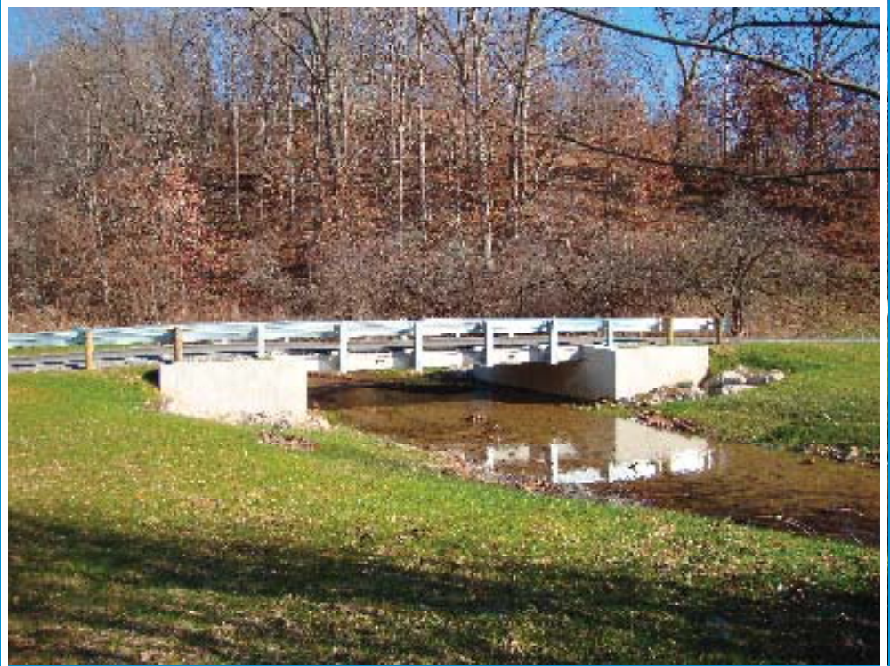
Picture above shows Sugar Camp-Jackson Fork Road Bridge completed.
